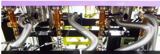
Figure 4: Photo of the outer windows installed on the FPCs.
