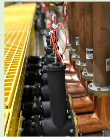
Bias tees installed in the tunnel for HWRs.
