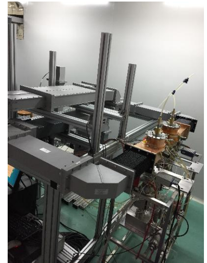
On site installation
