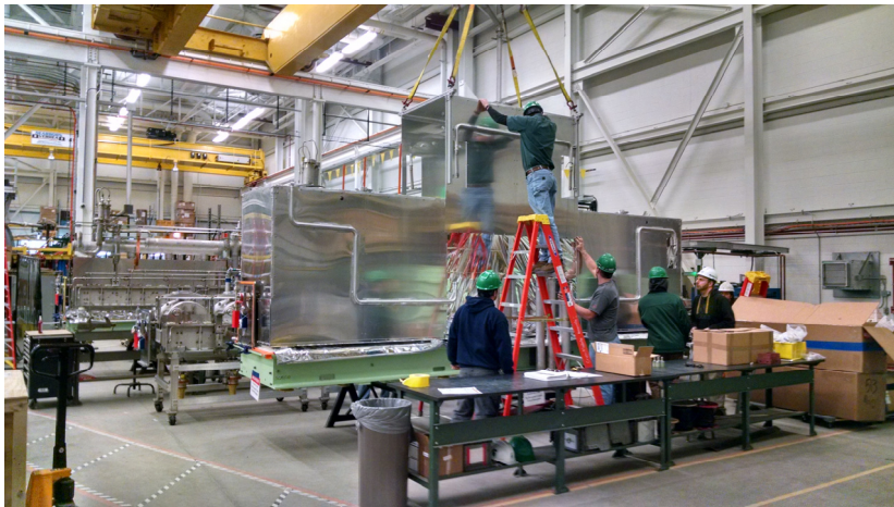
Thermal Shield Installed
