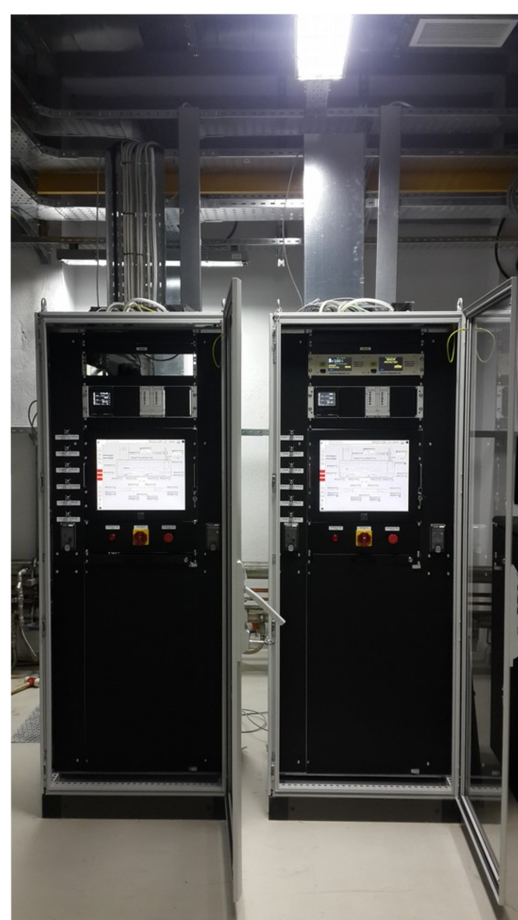
Control cabinets of TARLA Cryomodules
