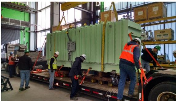
Figure 12:  $\beta=0.53$  cryomodule being loaded onto low deck truck. The cryomodule is secured to the deck of low boy truck by ratchet straps prior to rigging removal.
