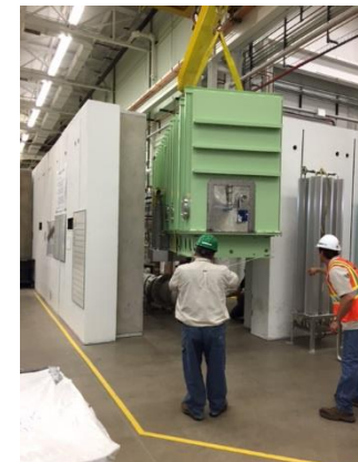
Installation of cryomodule into test bunkers
