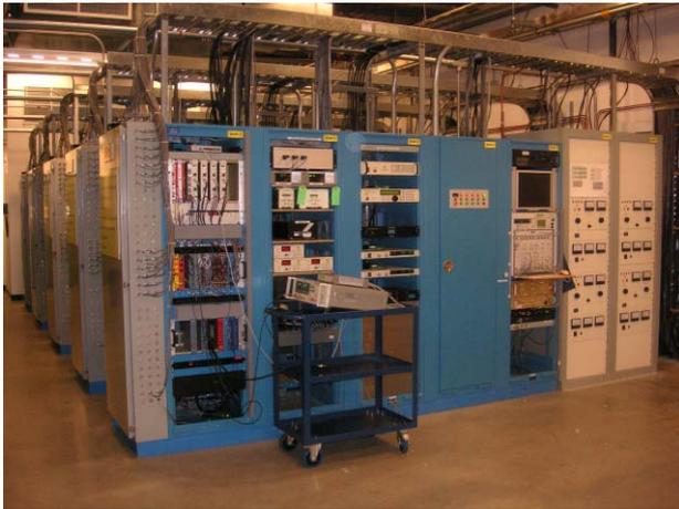
Figure 1: Layout of RF Amplifiers for Medium Beta Linac in the Power Supply Room
