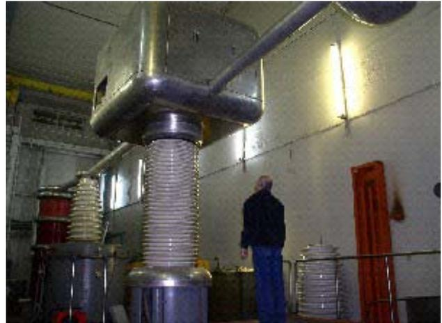
Figure 2: View of HV devices: there is the ion source supply system dome on the white insulate column at the first plan, then 400kV pulse transformer is seen, the diode stabilizer rack has been placed after the latter.
