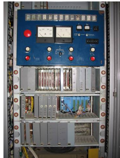
Figure 3: ADAM-500/485 in the control cabinet of SCS.
