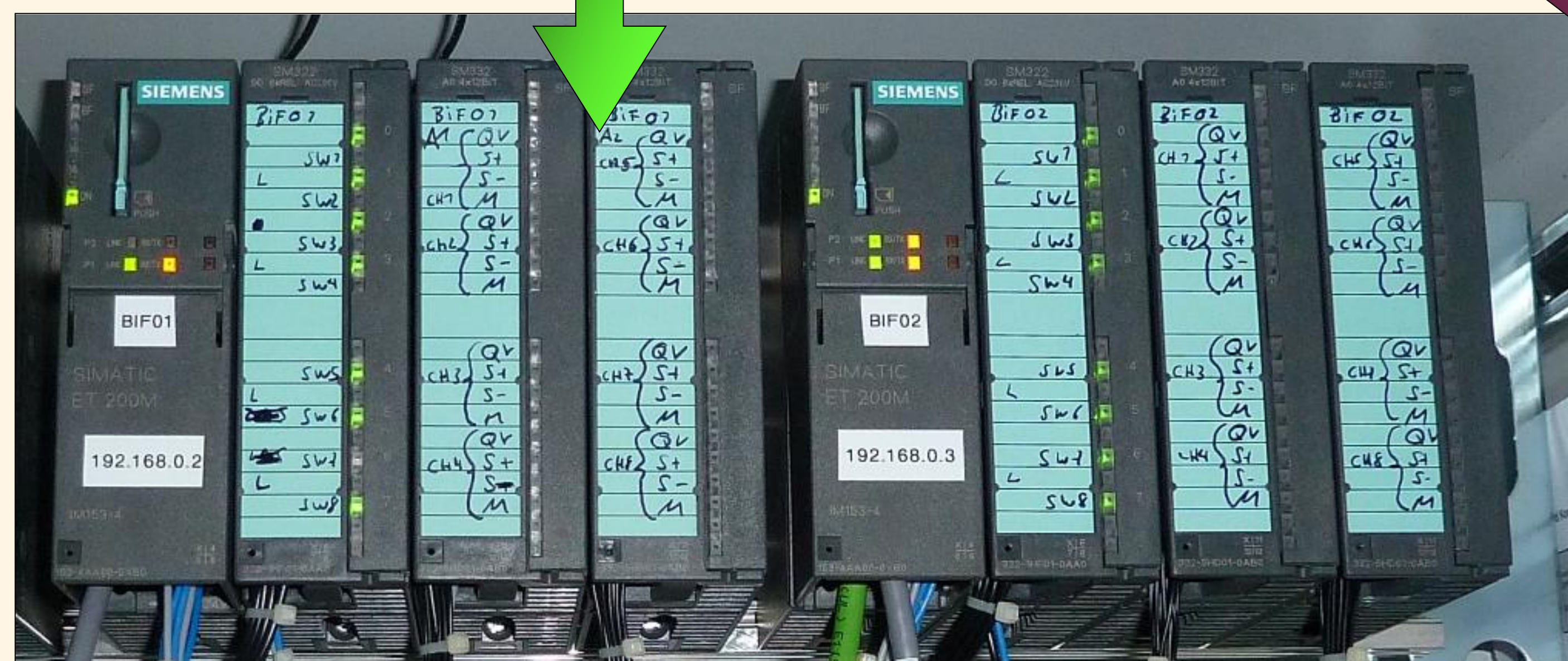
satellite installation in radiation-safe area near experiment to control two BIF monitors: contains two sets of: satellite controller, relay module, DAC module (2x)
