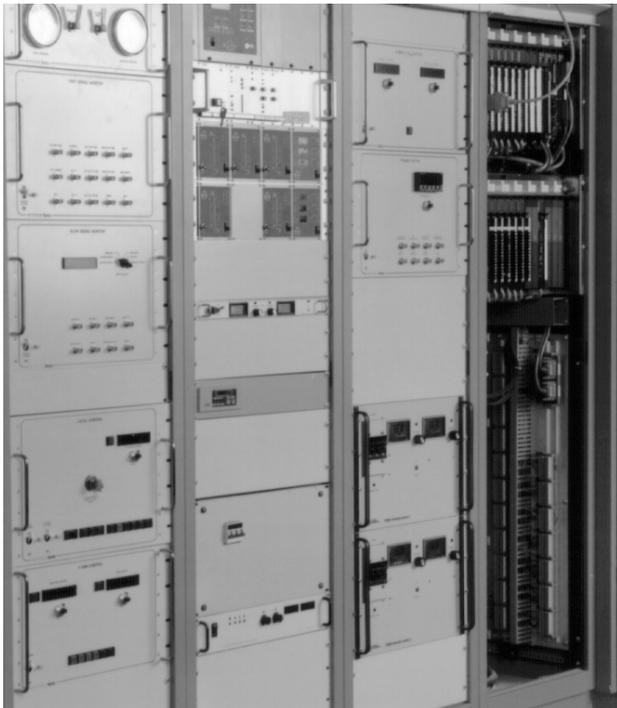
**Fig. 6.** Local controls and power supply rack. The PLC also resides in this rack.
