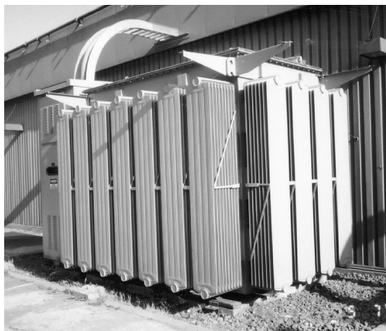
Figure 7: Power supply installation
