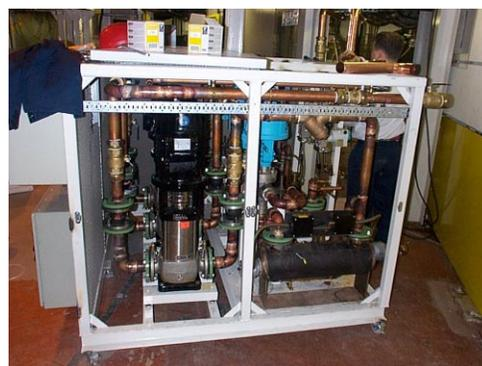
Figure 4. Cavity Water Control Station.
