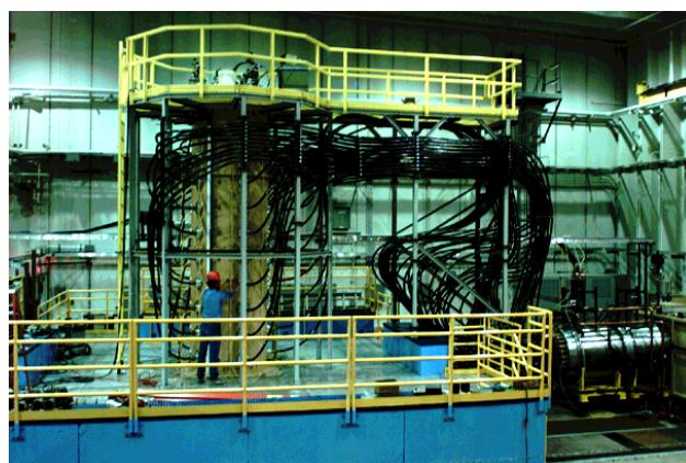
Figure 3. 2.5 MV RHEPP-II voltage adder
