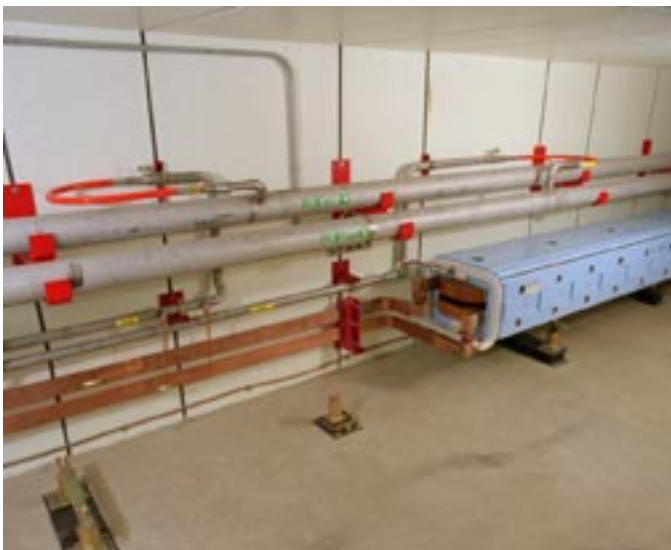
Figure 4. Prototype Q601 Hydraulic Cell Installation
