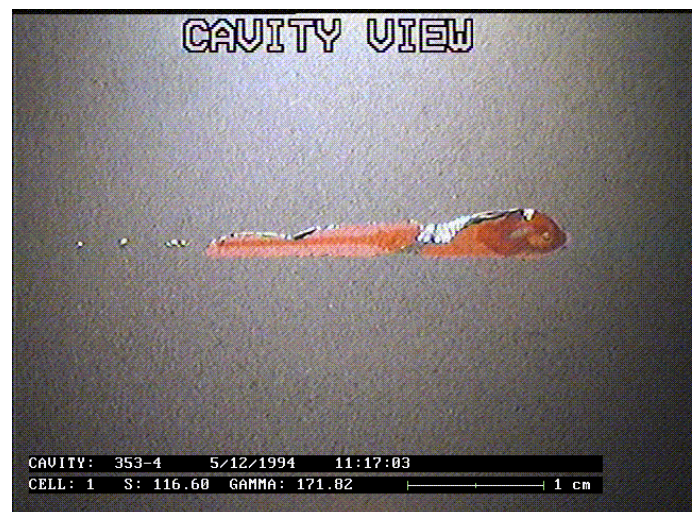
Fig.1: Major defect on the inner cavity surface (~2 cm).
