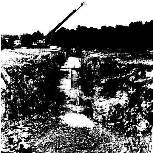
Figure 1. Excavation and foundation of the linac tunnel.
