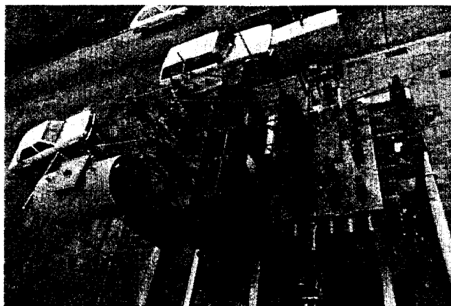
Fig. 1 Open air equipment PETRA I – power supply (SR)
