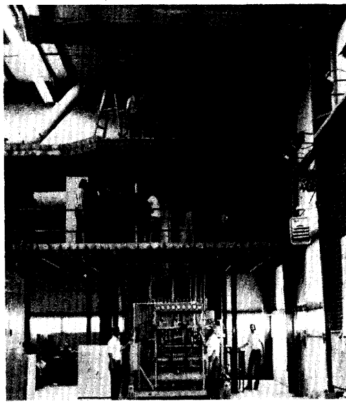
Cold Box and Turbine Oil Skid
