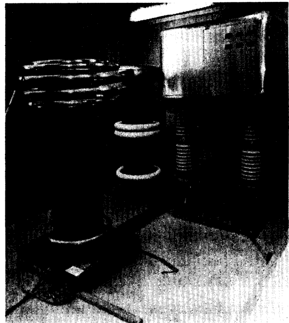
Figure 2. Power Supply, Isolation Transformer and Dome
