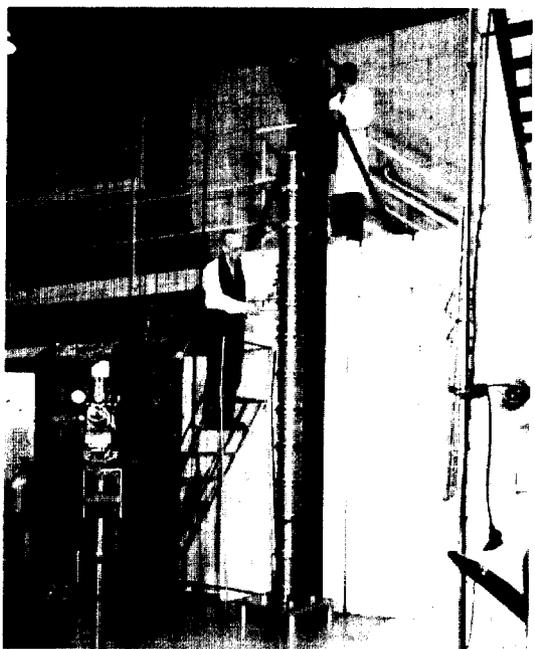
Fig. 2. The accelerator tube being assembled.
