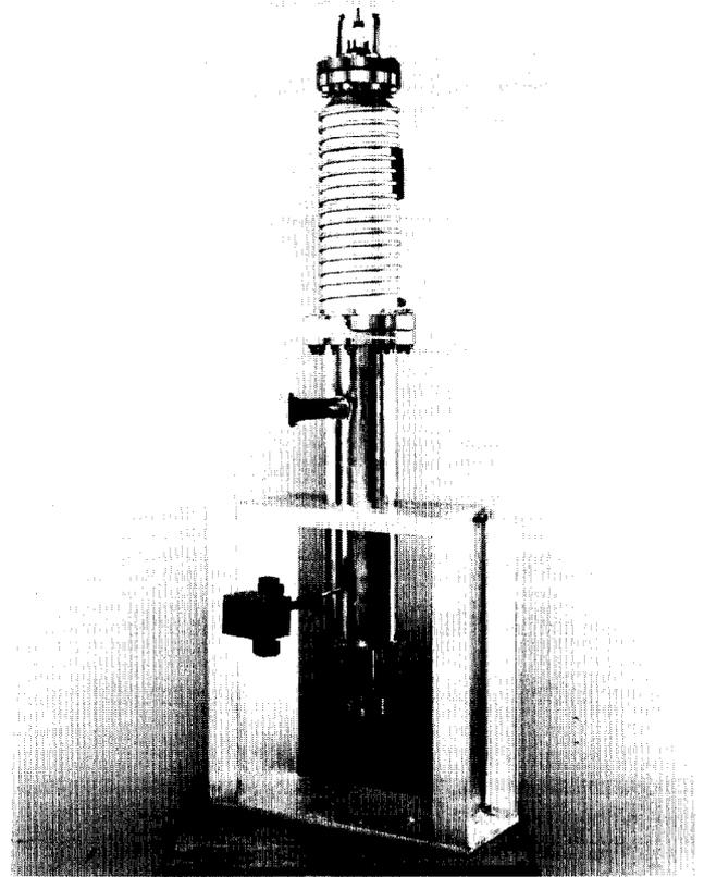
Fig. 4. N.R.C. Orbitron-type pump, 400  $\ell$ /s, with std. tube.
