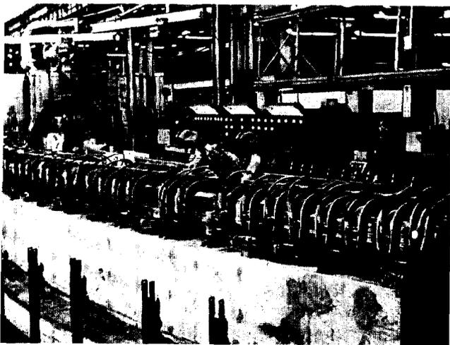
Fig. 4. Argonne ZGS Ring Magnet Coil Molding Fixture.
