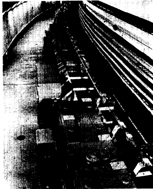
Figure 3. The Brookhaven AGS complete magnet system is shown in place in the ring tunnel. In the foreground is a 10 ft. straight section (with one of the rf accelerating stations); the back legs of the groups of magnets are alternated between positions inside and outside the orbit at these straight sections.
