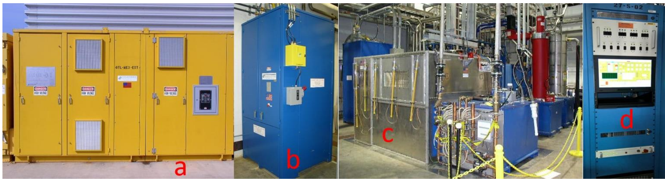
(a) 13.8 kVAC switch gear and magnetics, (b) six pulse-controlled rectifier unit, (c) high voltage enclosure and tank with a klystron (red) in background, (d) HVCM controller rack [3].
