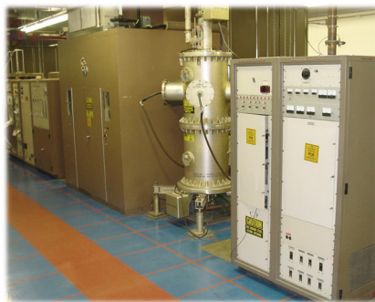
Hard-Tube Modulator & Triode Tube
