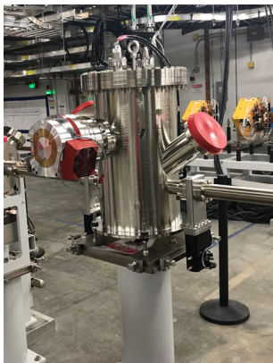
Carbon stripper installed to beamline
