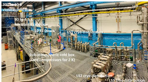
Figure 10: FRIB cryoplant operating at both 4.5 K and 2 K. Segmented distribution lines are connected to the refrigeration system with the U-tubes.
