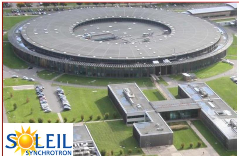
SOLEIL is the French synchrotron located on the "plateau" de Saclay" in Saint Aubin (Essonne) near Paris, both a large scale facility (storage ring of 354 meter circumference) and a research laboratory. Actually, there are 29 operational Beamlines (on 43 possible slots).
