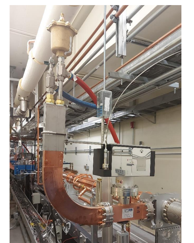
Figure 11 Vents installed on top of the RF Load
