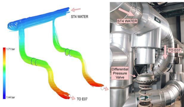
Figure 4: CFD of the ST4 water circuit. Details of pressure distribution in E07 inlet.
