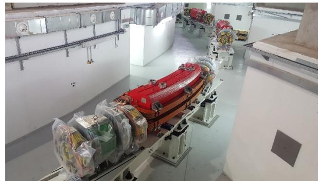
Figure 9: Magnets installed on Girder.
