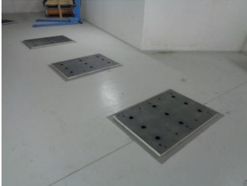
Figure 5: Girder Baseplates installed.
