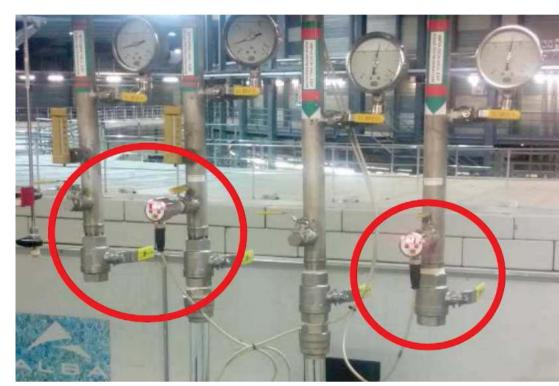
Flow data has been acquired using ultrasonic flowmeters and pressure sensors.
