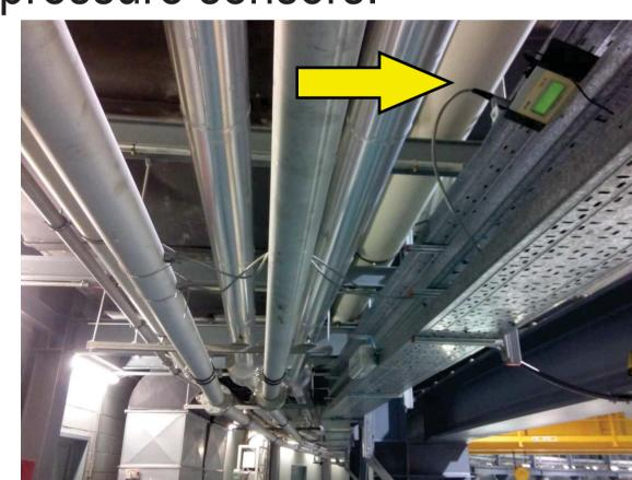
EA Ring feeds 7 out of the 32 beamlines (the capacity of ALBA), at a 8,6 bar and flowing at  $27 \ m^3/h$ .
