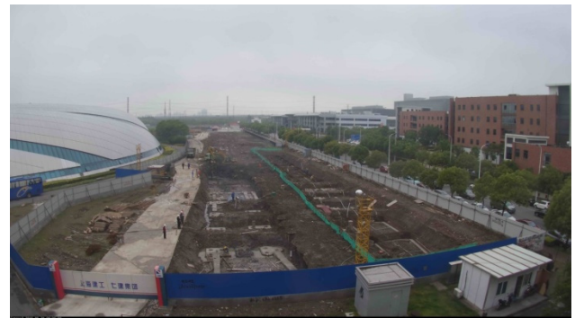
Figure 9: SXFEL construction site at 9:00 A.M. on May 28, 2015.
