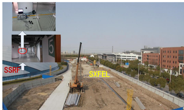
Figure 2: Test site on the floor of Experimental Hall.
