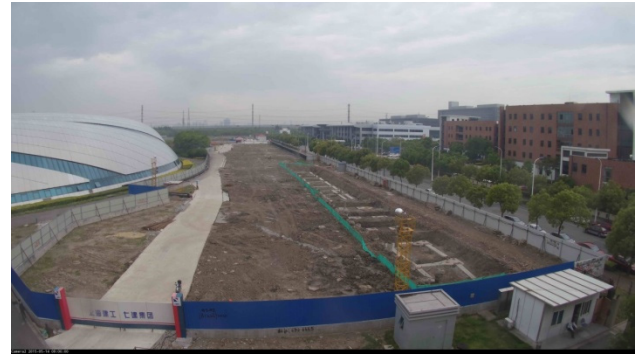
Figure 8: SXFEL construction site at 9:00 A.M. on May 14, 2015.
