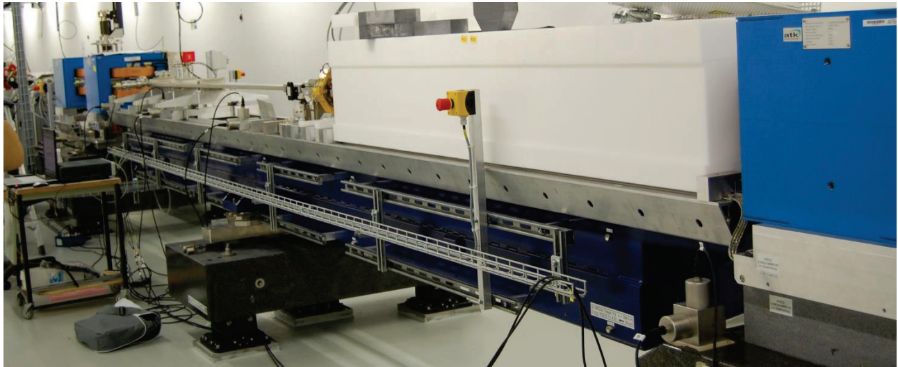
Figure 9 Vibration measurement on SwissFEL BC2
