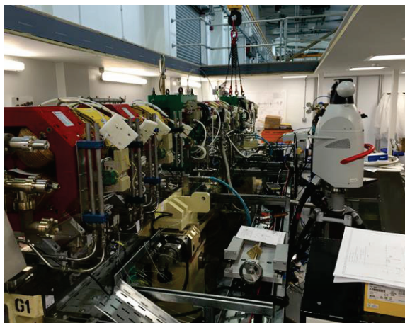
Figure 2: Completed Girder 1 in the assembly room.
