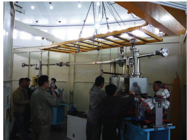
Figure 5: Installing a subsystem.
