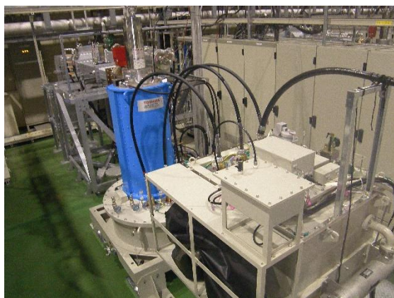
Figure 11: 972-MHz klystron station.
