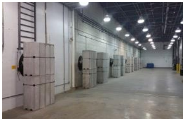
Figure 9: Klystron gallery after the completion of the chase insert activity.
