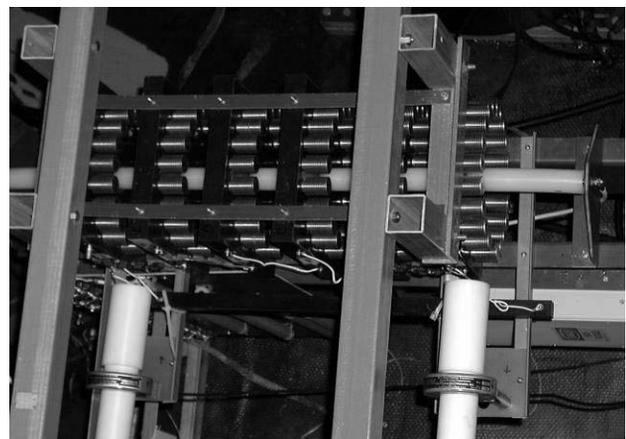
Figure 1: 60Kv 20A-50A switch as installed at the base of the IPNS ion source.
