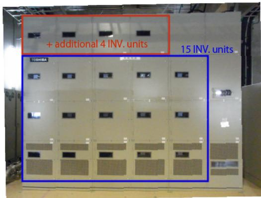
Figure 2: Anode power supply with 19 inverter units
