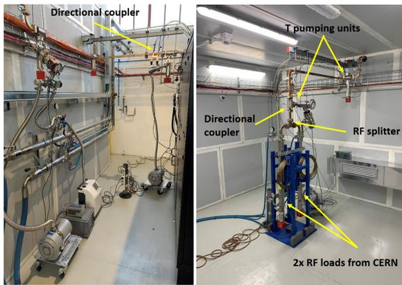
Figure 2: Pictures of the waveguide network in the klystron area (left) and inside the bunker (right).
