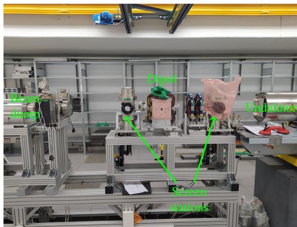
Figure 4: In the straight section all support structures for the beam line elements as well as the two screen stations and the dipole to separate electron and THz beam are installed and aligned. The bellows and beam pipes connecting the undulator and the beam dump are ready for installation. The dispersive section with the high power beam dump is currently in production.
