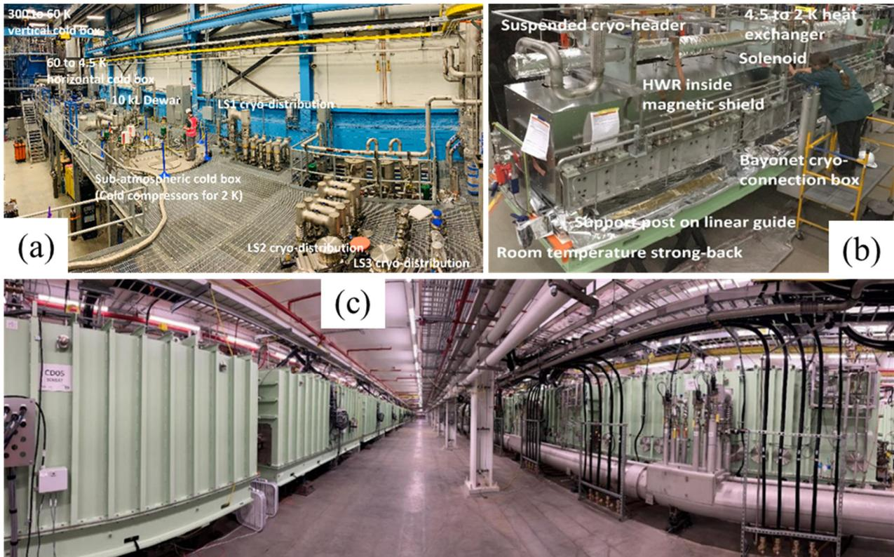
Figure 2: (a) FRIB helium refrigeration plant. (b) Partially-assembled FRIB  $\beta = 0.53$  cryomodule. (c) FRIB driver linac tunnel, about 10 m underground (left: LS2; right: LS1).
