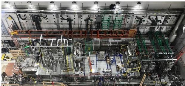
Figure 4: FRIB Target Hall, including the production target, beam dump, and wedge systems, with vessels and radiation shielding.
