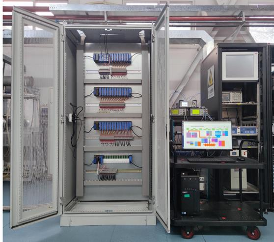
Figure 2: PLC cabinet of the DAQ system.
