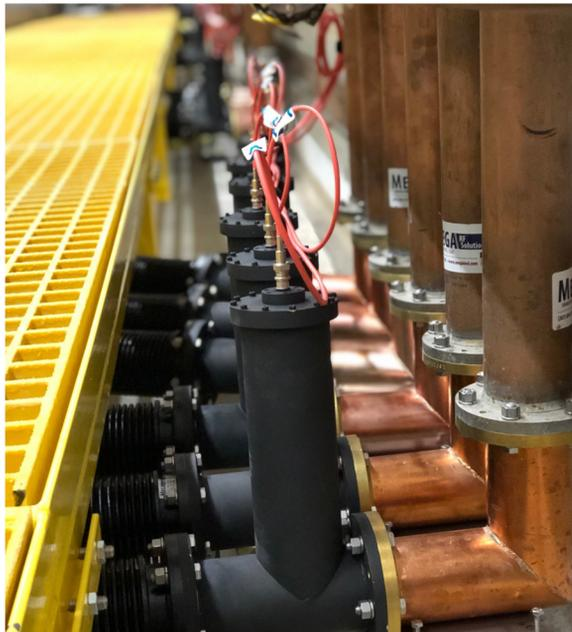
Figure 4: Mega bias tees installed in FRIB.
