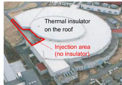
Figure 2: Photograph of the PF Light Source Building. A red frame area is the injection area including a part of the transport line and has no thermal insulator on the roof.
