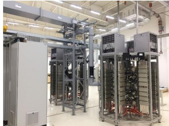
Figure 1: SSA towers of the storage ring RF plant.
