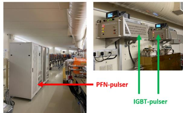
Figure 6: Comparison of the spatial occupation of the PFN pulser and the IGBT pulser.
